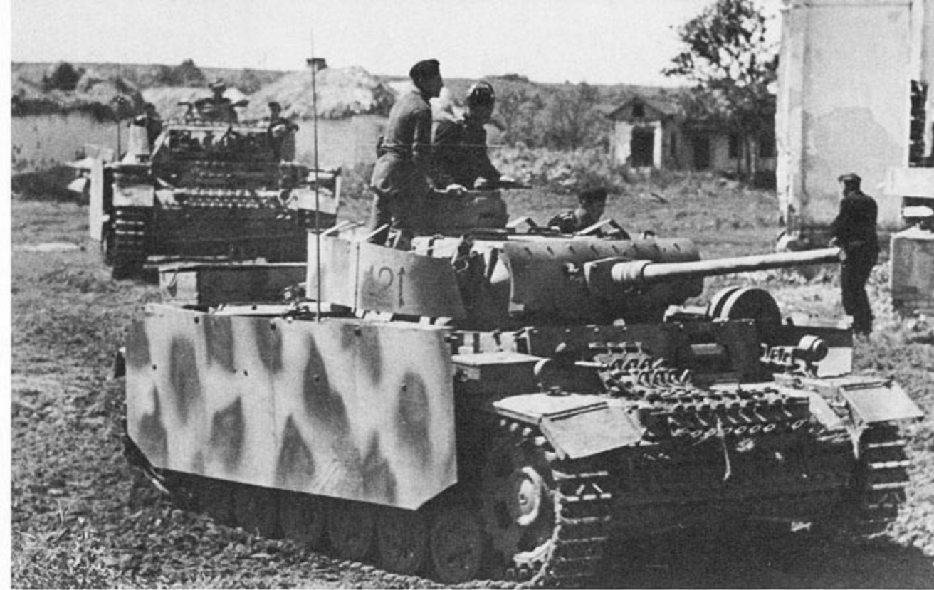
A PzKpfw III Ausf M, followed by an Ausf J, advances through a Russian village during 1943. The Ausf M has an earlier style headlight in place of the starboard Bosch light. The camouflage is Dark Yellow oversprayed with patterns of Olive Green outlined in Red Brown and the turret numbers are in Red.
