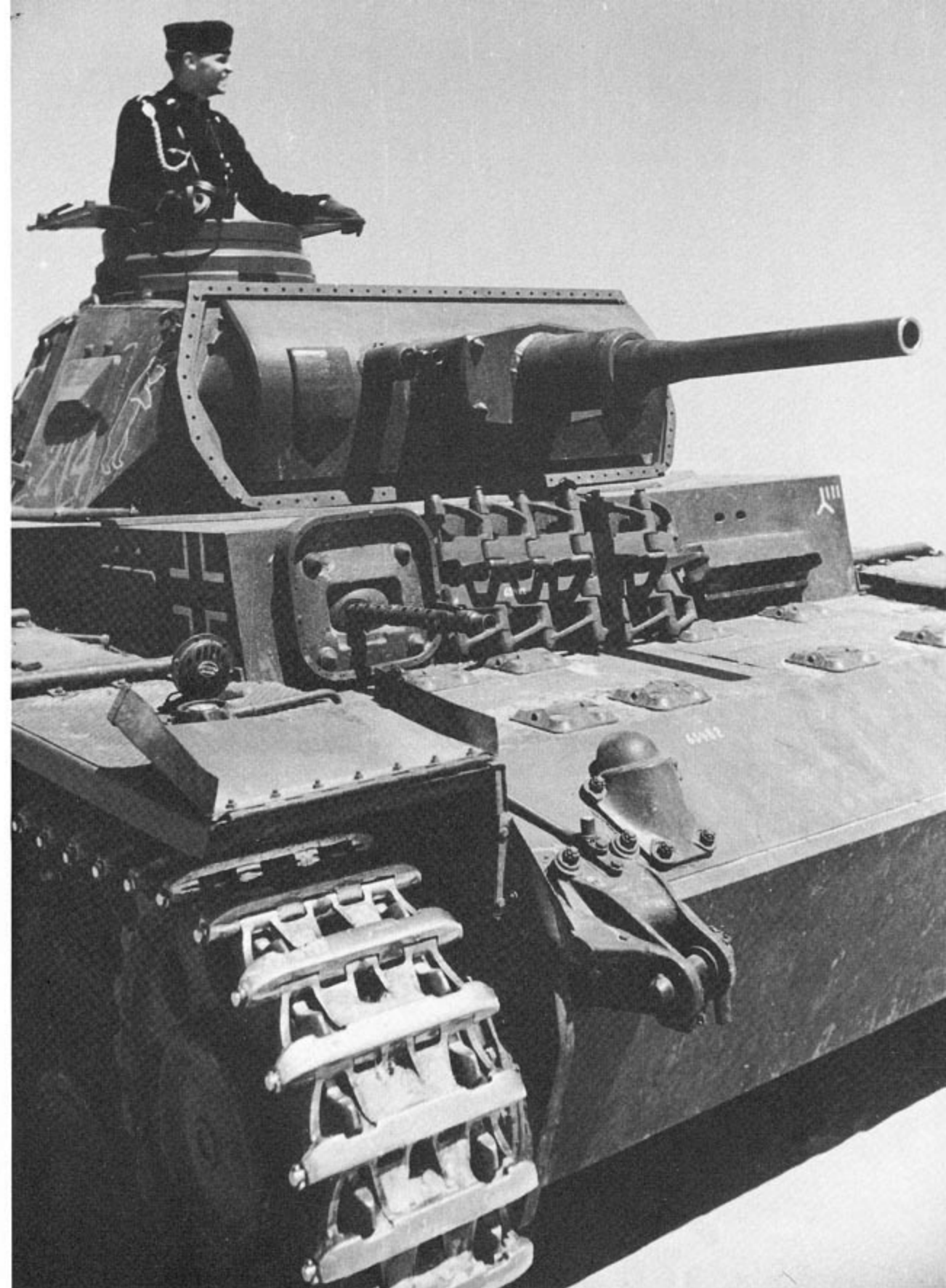
When the invasion of England (OPERATION SEA LION) was cancelled the majority of Tauchpanzer III's were modified as wading tanks. This wading tank is attached to 4.PzDiv for training. The frame around the turret front was the mounting frame for the gun mantlet waterproof fabric cover.
