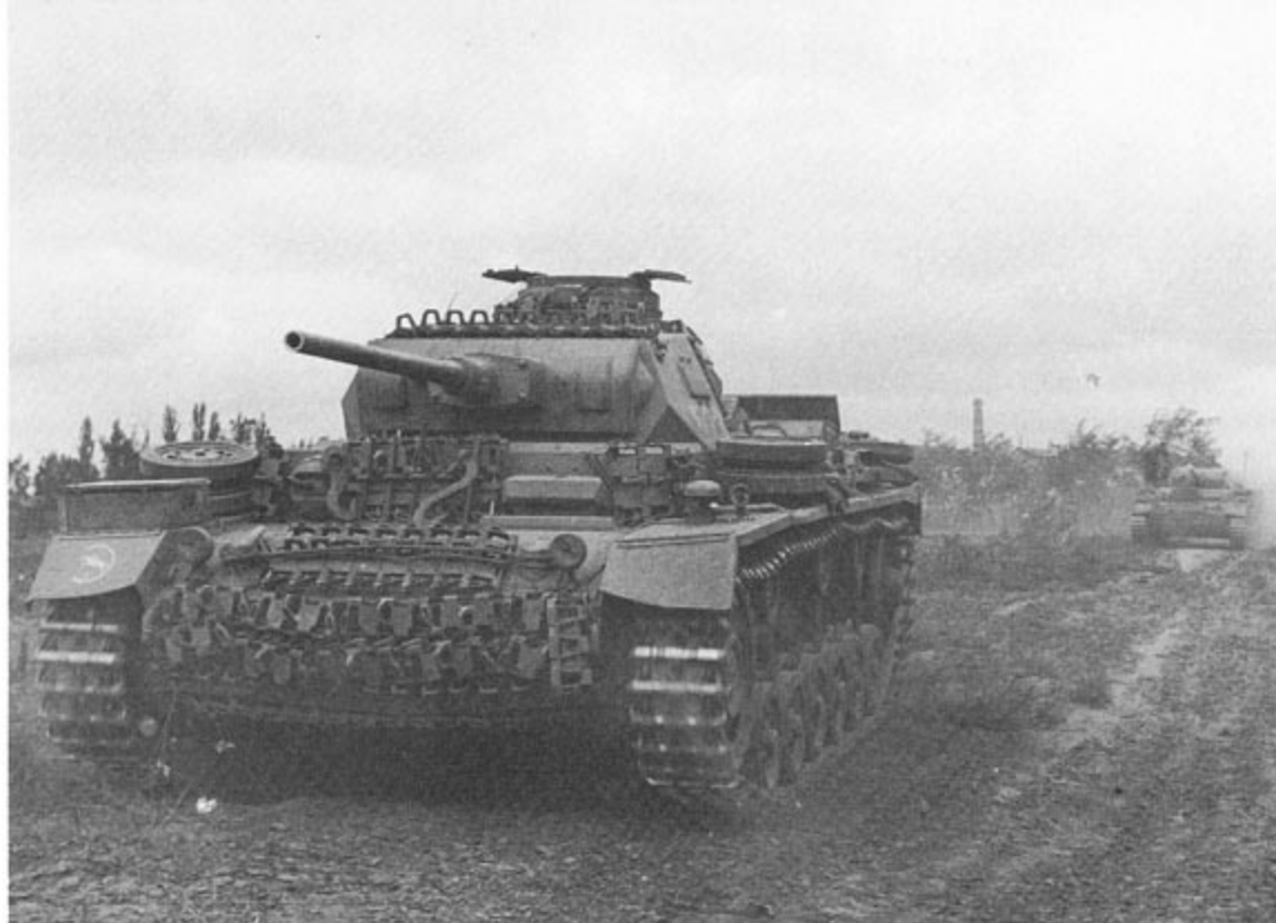
PzKpfw III Ausf Js of 24.PzDiv advance toward Stalingrad. The crew has added extra track links to the turret roof as well as the superstructure and hull front. The division sign on the starboard fender and the outline Panzer unit rhomboid tactical sign on the gun recoil tube are in White.
