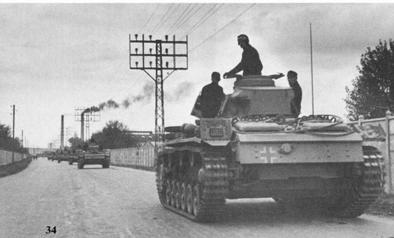
A column of late production PzKpfw III Ausf Ls advance through a town in southern France. The cutout in the left rear mudguard was to allow installation of a Notek blackout tail light.
