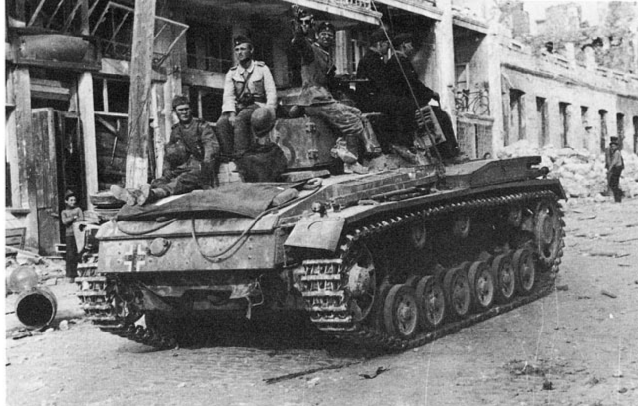
German infantry catch a ride on the back of a PzKpfw III Ausf L as it passes through a Russian town during the Spring of 1943. The large national flag on the rear deck was used as an aerial recognition aid. This tank is painted overall Dark Yellow, the turret numbers are in Red and the tactical signs on the tailplate are in White.
