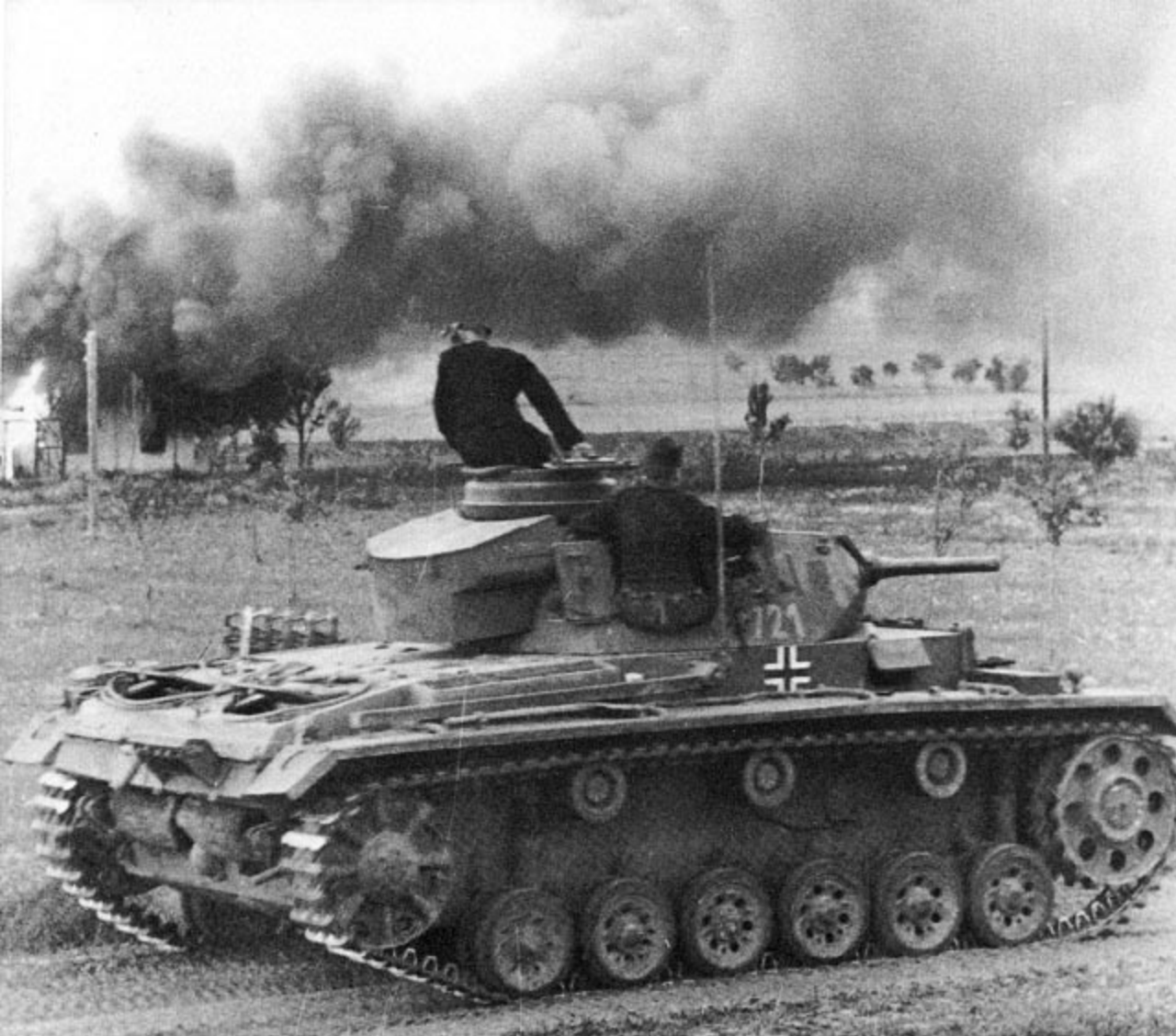
(Above) An overall Dark Gray PzKpfw III Ausf G of PzRgt 31, 5.PzDiv passes a burning building during the invasion of Russia. The turret stowage box on the back of the turret became a standard feature on later variants and was often retrofitted to earlier models.
