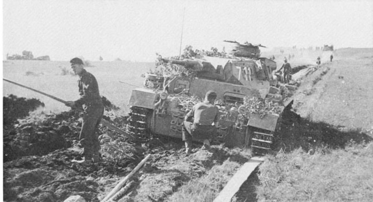
Crewmen work to free a bogged down PzKpfw III Ausf H of 1.PzDiv on a dirt road in Russia during early 1942. The superstructure front carries applique armor plate with cutouts for the driver's visor and hull MG mount. This vehicle is painted in the African camouflage scheme of Yellow Brown.
