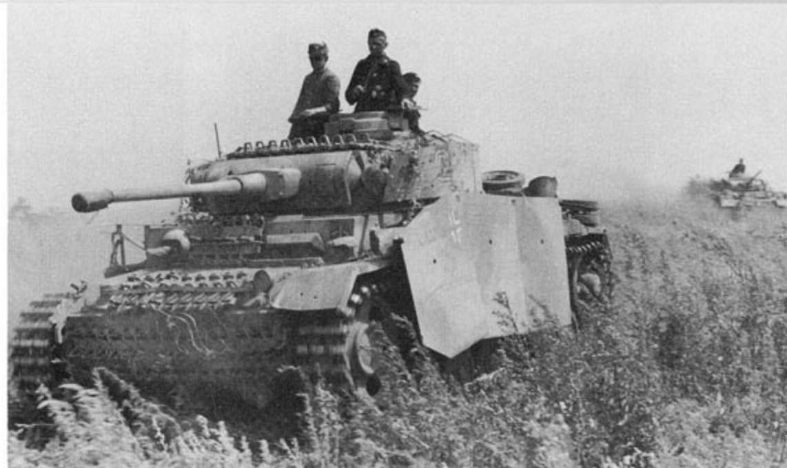
Late production PzKpfw III Ausf Js, and rebuilt earlier variants, were fitted with thin armor skirts for protection against shaped charge projectiles. This Ausf J of 20.PzDiv in Russia is camouflaged in Dark Yellow over-sprayed with broad areas of Olive Green with the division sign in Yellow Ochre against a patch of the Dark Gray.
