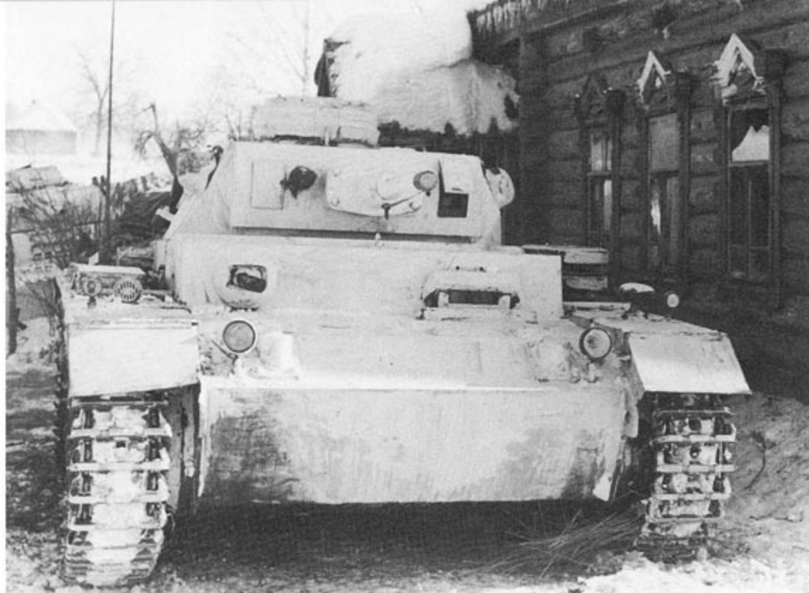
This snow camouflaged PzKpfw III Ausf J has the port vision flap on the mantlet open and has dust covers on all the weapons. The White temporary camouflage was washable and quickly wore off in action.
